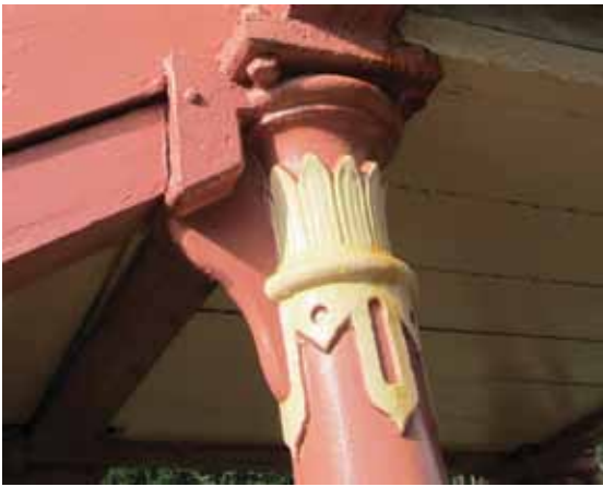
Hagley Station Footbridge
