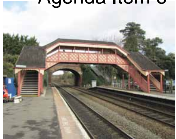
Hagley Station Footbridge
